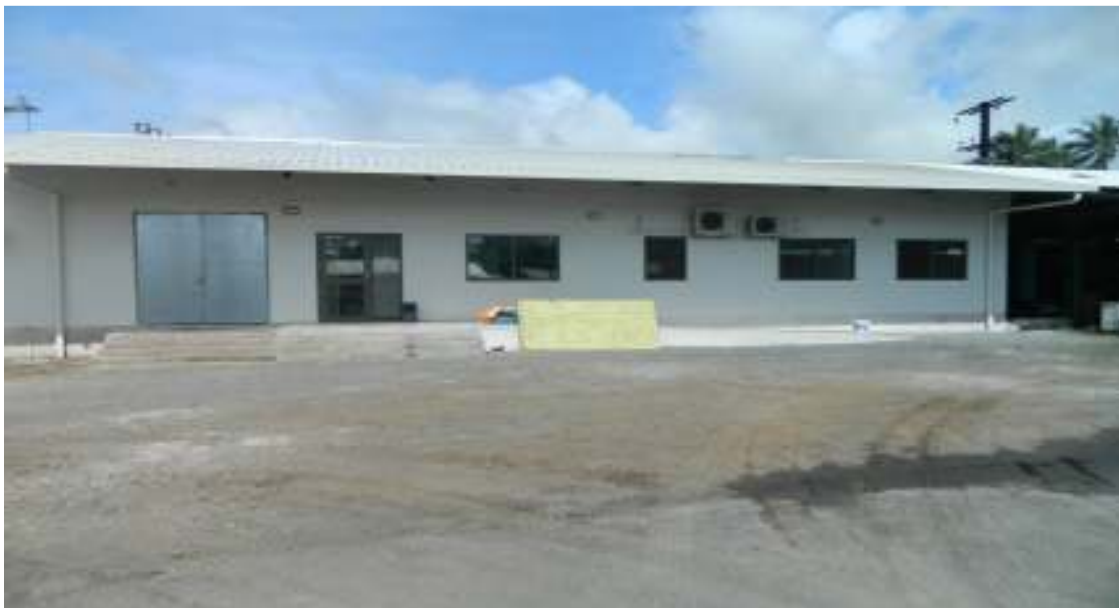
Salelologa Substation Building
