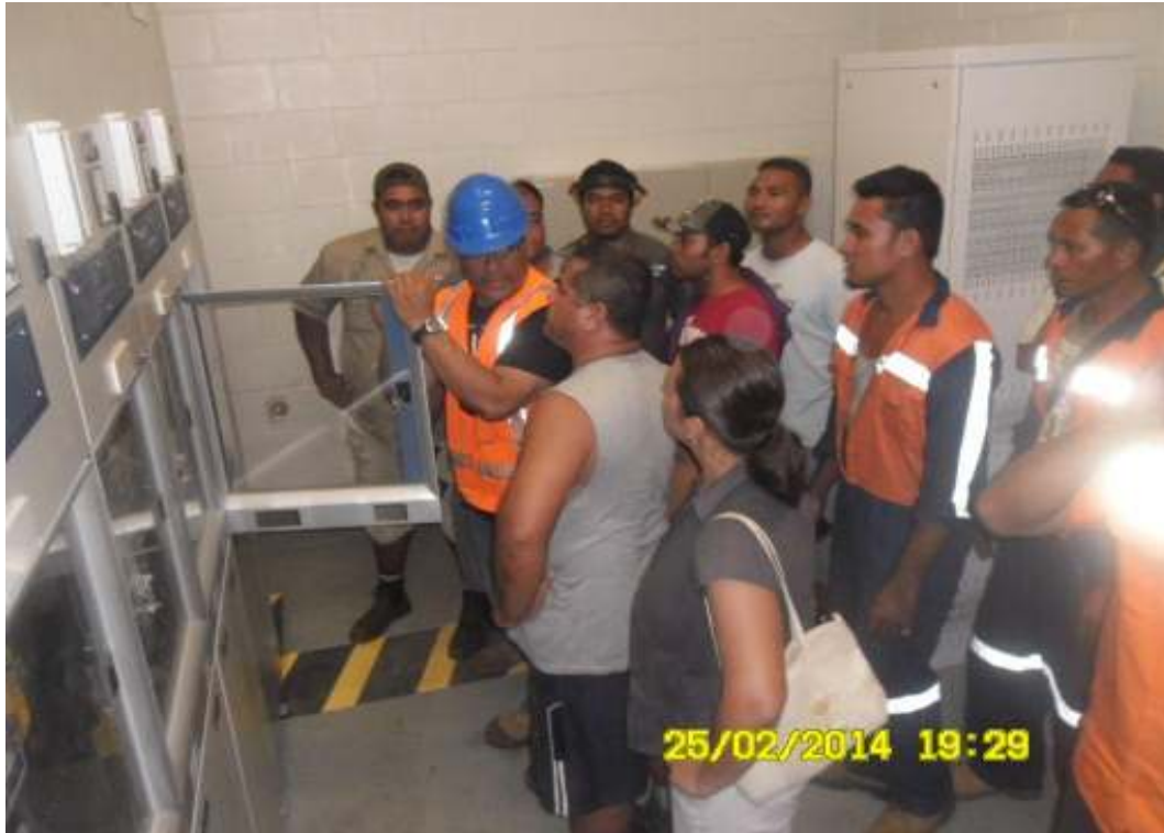
EPC Engineer and IPES member Tupai Mau Simanu (in blue helmet) conducting the training for EPC workers for the new switchgear
