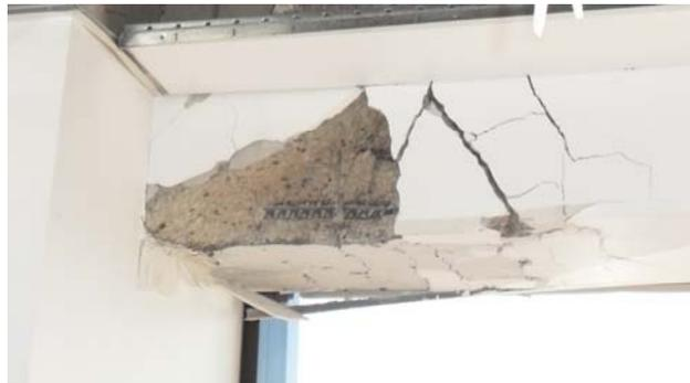
*Figure 1: An energy absorbing (ductile) beam hinge in a reinforced concrete building after an earthquake. As these ductile elements yield they absorb energy without loss of strength that would lead to collapse of the building. While some of the cover has fallen off, none of the reinforcing has broken, and the concrete inside the reinforcing cage is intact, so this beam can still carry load.*
