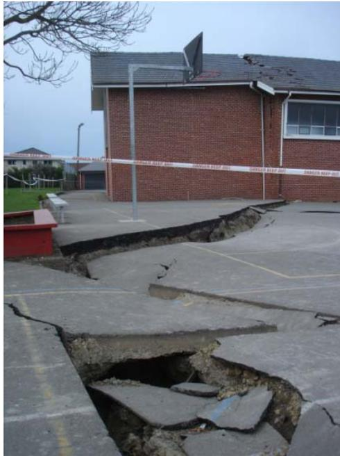
*Figure 8 Lateral spread crack running through the courtyard and building at St. Paul's church, Dallington, Christchurch, New Zealand (September 2010)<sup>6</sup>*
