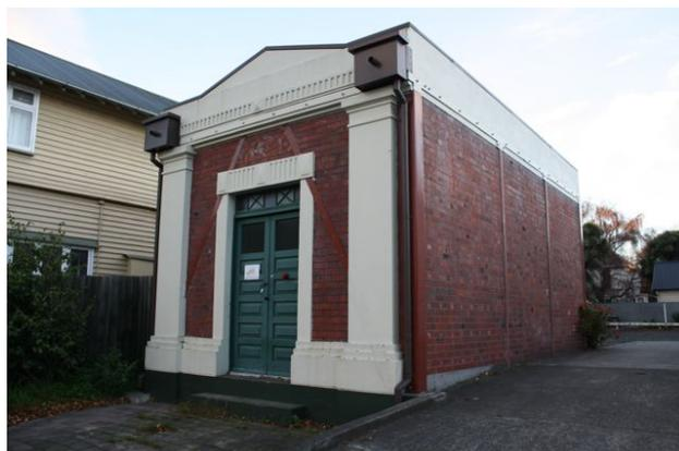
*Figure 9: Orion Local Substation. Constructed in unreinforced brick masonry that has been strengthened with a steel perimeter frame (Photo Win Clark)*
